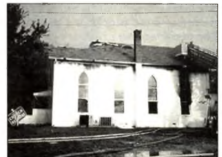
Eight fire stations battled for eight hours to fight the fire that eventually destroyed Clayton, Ind., Church of the Nazarene. Damage to the 100-year-old-plus building was estimated at a million dollars.
