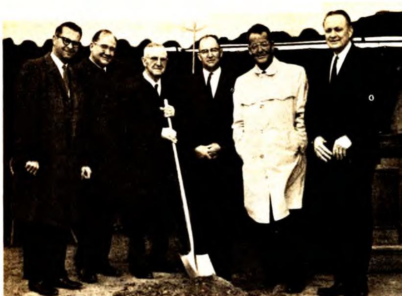
LAUNCHING A BUILDING PROJECT, L. R. Rice (with shovel), a member of Greeley (Colorado) First Church for forty-two years, turns over the first spade of dirt. The ground-breaking marked the start of a $100,000 church and educational building. From left are Rev. Earl B. Wheeler, pastor; Wilson Rice, L. R. Rice, Harold and Bill Rice, and Rev. E. L. Cornelison, Colorado District superintendent. Wilson, Harold, and Bill are sons of L. R. Rice.
