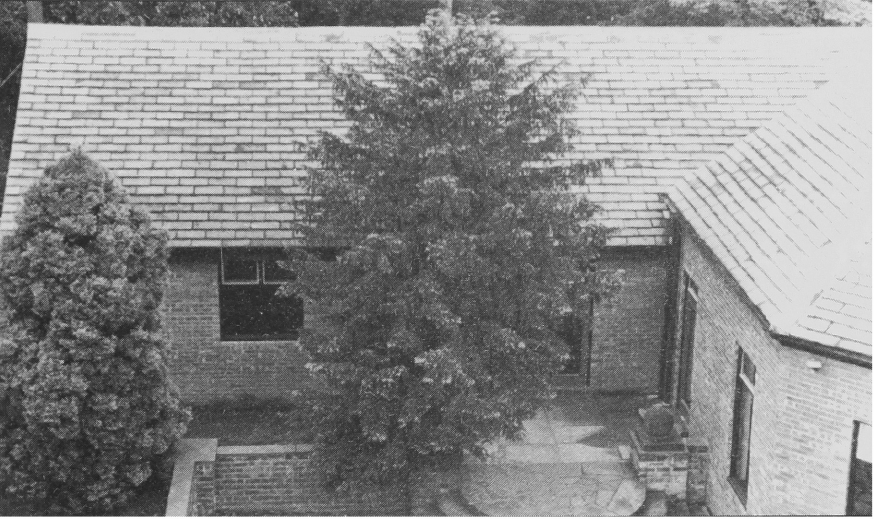
Photo No 40 New Dining Hall adjoining the Chapel
