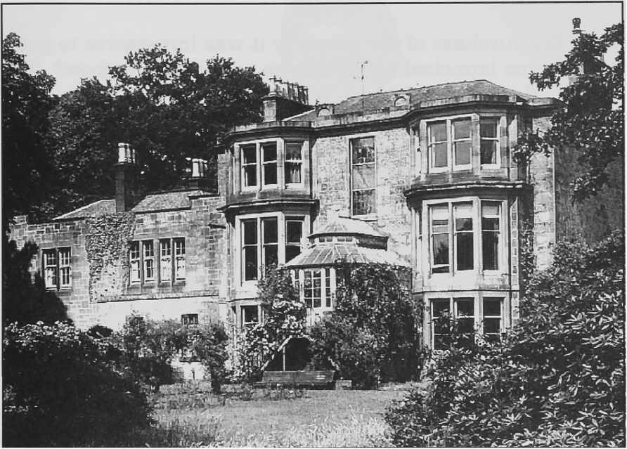
Photo No 4 West Hurllet House, Barrhead, Glasgow
