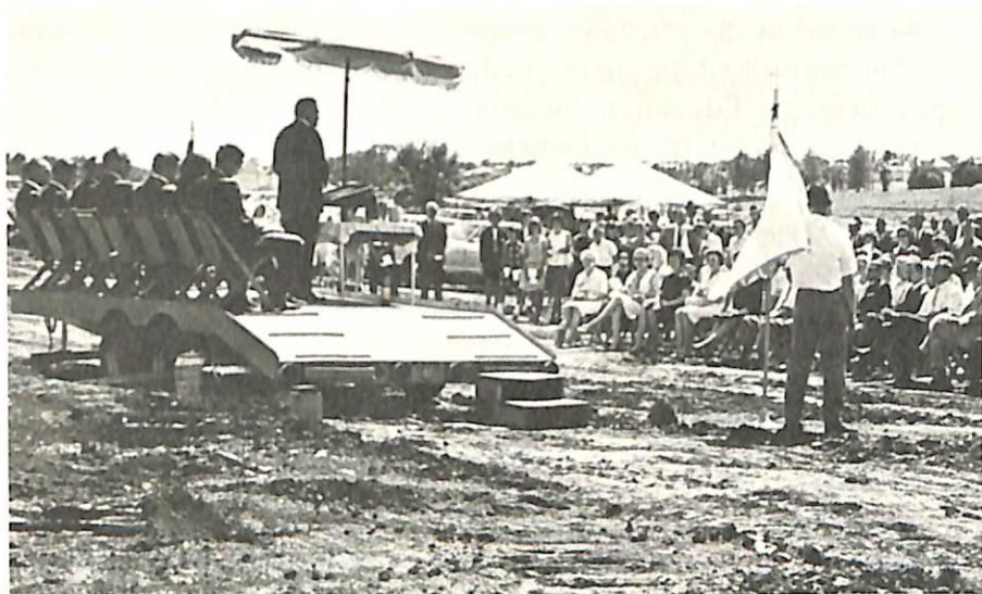
Wilson R. Lanpher, first chairman of the Board of Trustees, addresses the groundbreaking crowd in 1967.
