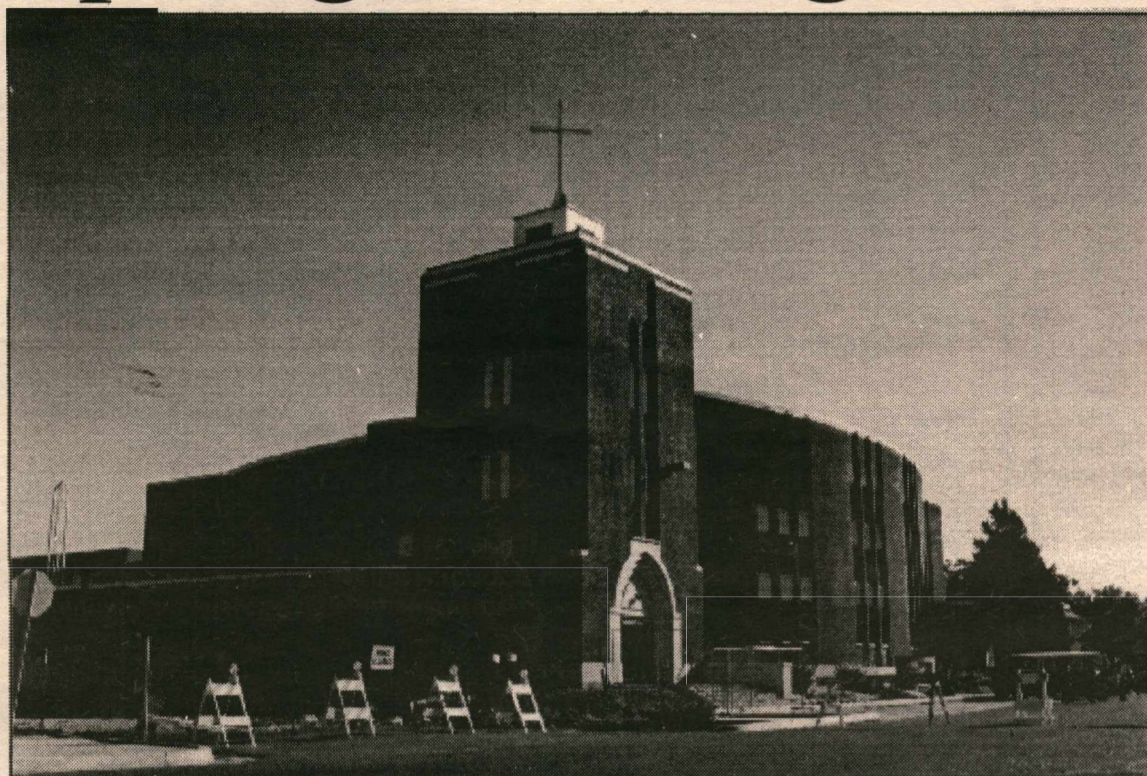
College Church under construction
